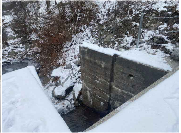
November 2021 – Right wall of Outlet Flume
