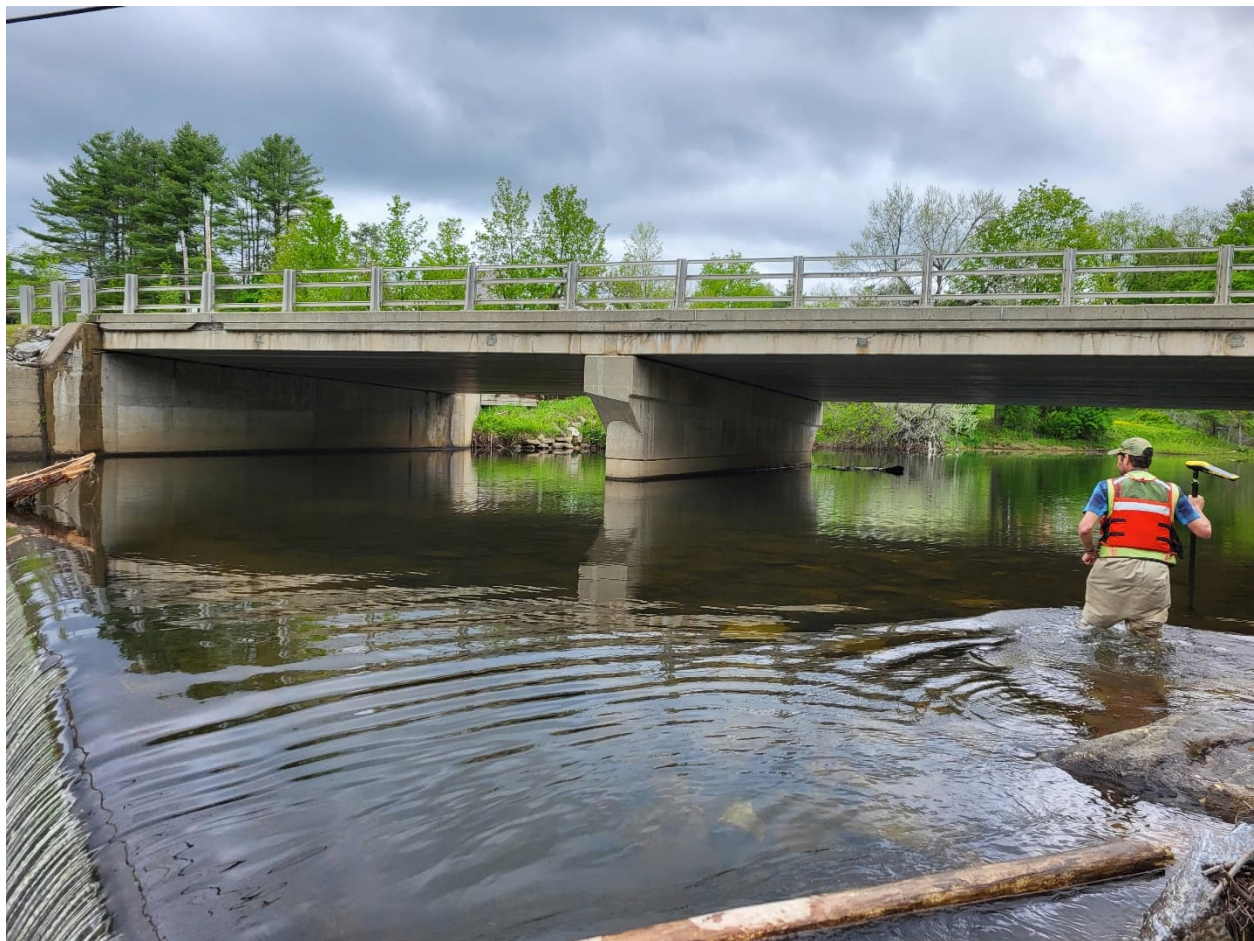
Figure 5: VT Route 11 Bridge (Looking Upstream from the Dam)
