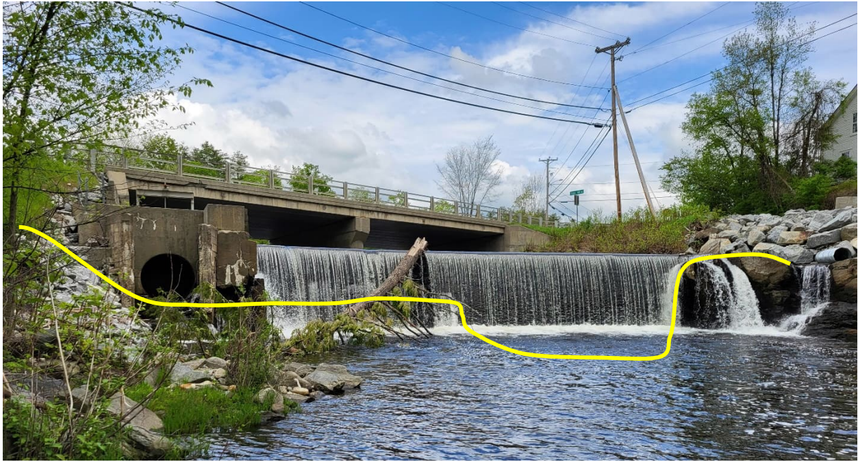
Figure 3: Williams Dam (Looking Upstream) and the Potential Underlying Bedrock Channel Section (Yellow Line)
